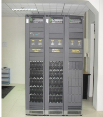
Gambar 3.25 Rectifier Cabinet Forza Power One [13]
