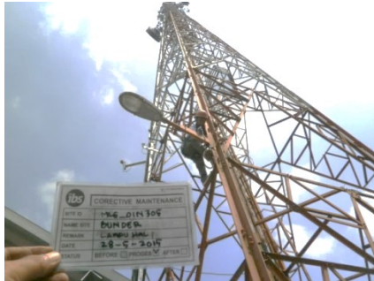
Gambar 4.30 Proses penggantian lampu tower
