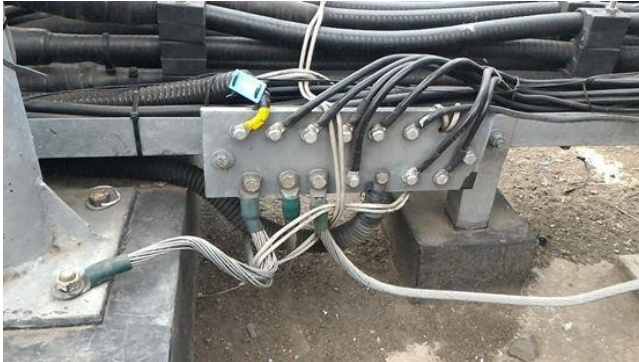
Gambar 4.13 RF Grounding
